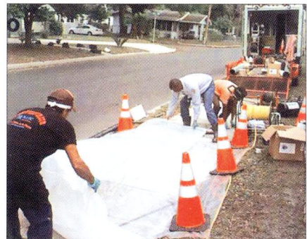
Using spot repair, crews are able to work in a small site area and reduce disruption associated with open-cut.
