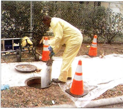
After cleaning and inspecting the pipe, the liners are lowered into a manhole and pulled into place.
