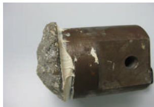
Concrete Pulled Out @ 464 psi.
